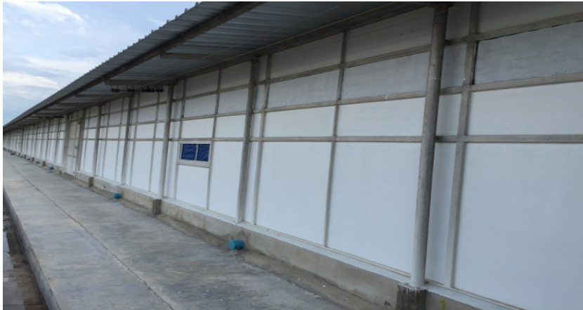
Figure 2. The natural lighting control house
